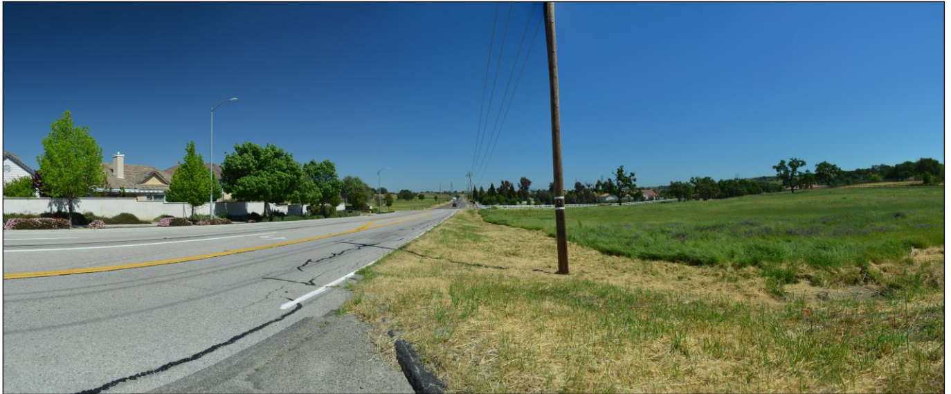
IOP C2 is looking northwest toward the power line route alternative along Creston Road. Photograph taken April 25, 2019.
